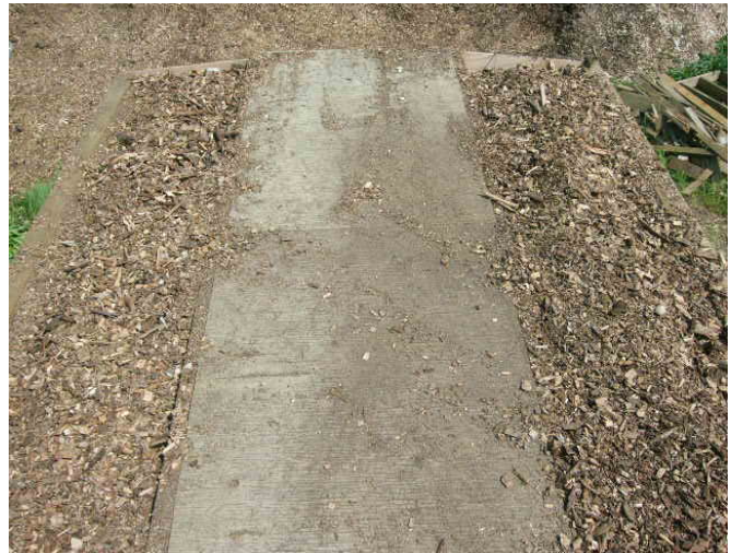
Fig. 3. Top view of a biofilter unit showing the two chambers filled with medium on alternate sides of a central plenum. There was no roof covering the unit.
